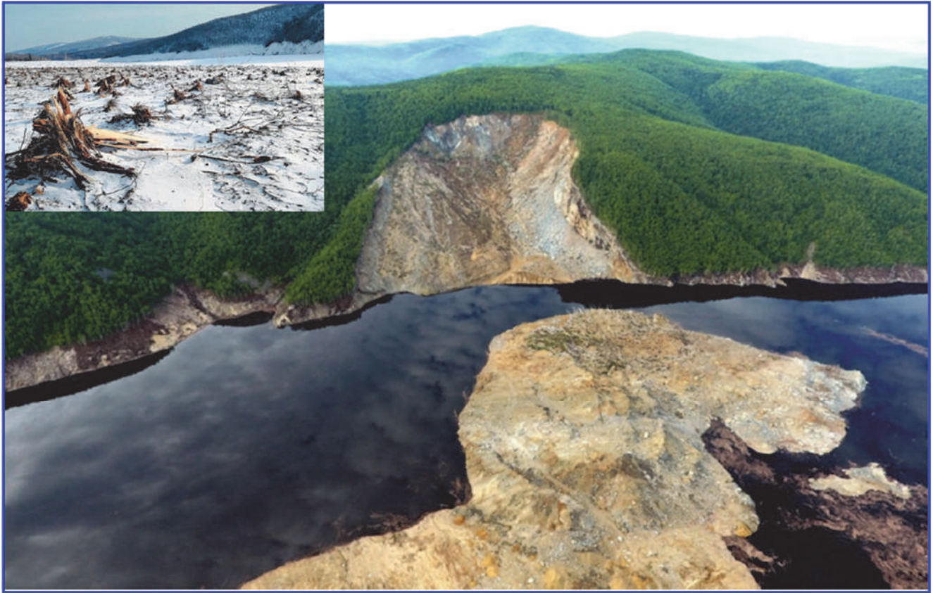
Fig. 15 General view of the landslide scar on the southern bank of the Bureya water reservoir and the body of the landslide with a passage, initially made 1 February 2019 and then extended by the spring flood in April-May 2019. The top left panel shows damaged stumps and exposed tree roots on the gentle coastal slope directly opposite the landslide on the northern bank of the Bureya river (Figs.3 and 9 in Gusiakov and Makhinov 2020)
