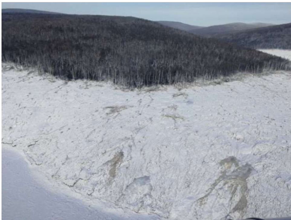
Fig. 2 The area on the right (northern) bank of the Bureya reservoir near the mouth of the Sredniy Sandar river. Note the evident trim line, below which vegetation and soil cover have been completely removed by the upslope water flow and the gullies produced on the steep coastal slope by backwash currents. Photo by A. Makhinov taken on 25.12.2018 from a helicopter MI-8
